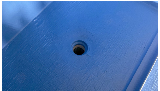
Pic 5. Protect your puddle flange with an appropriate membrane
