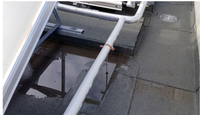
Pic 2. If ignored, ponding will damage the most robust membranes
