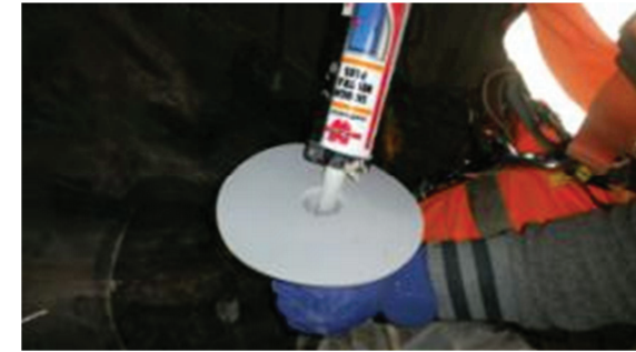
3. Fill the collar with swellable sealant
