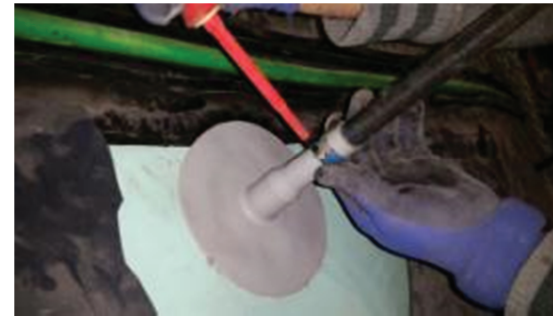
5. Install stainless steel clamp
