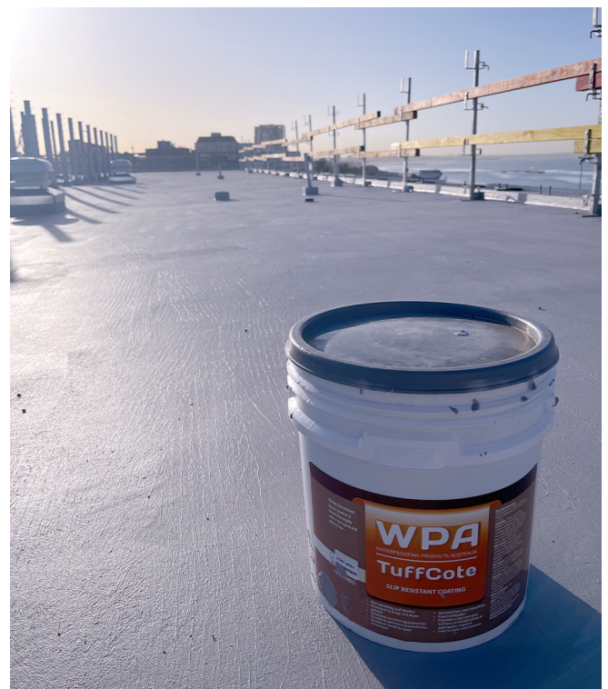
Pic 6. A coat of primer and a flexible membrane can go a long way
