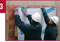
Peel back the top part of the silicone release film. Adhere COLPHENE 3000 to the substrate, making sure the membrane is well aligned.
