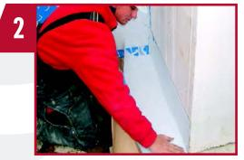
Install a reinforcement strip membrane centered on the corner of all interior and exterior foundation angles.
