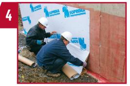
Gradually peel back the remaining silicone release film, making sure the membrane is completely adhered. The use of a hand roller is required to remove air pockets.
