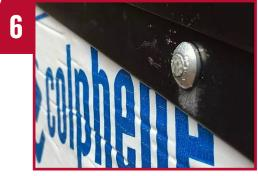
Use a pressure seal termination barre with a bead of SOPRAMASTIC / SOPRAMASTIC ALU to seal the membrane termination.
