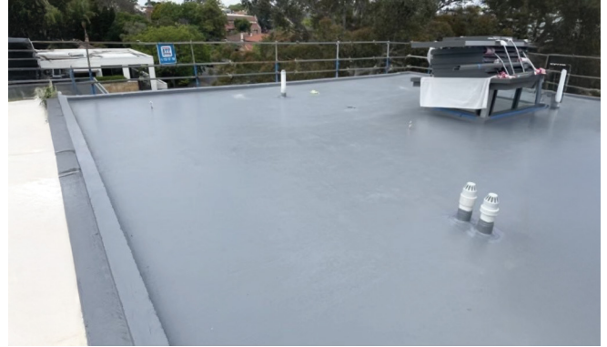
Pic 4. Substrate is smooth with no protrusions
