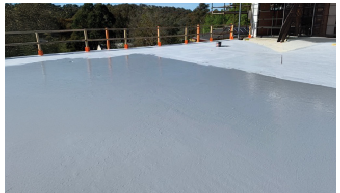
Pic 6. Free from voids and formwork distortions
