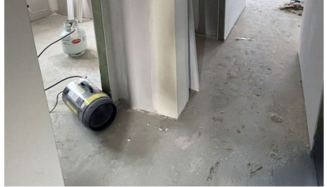
Pic 3. Industrial heater used in minus temperatures to assist dry/cure membrane
