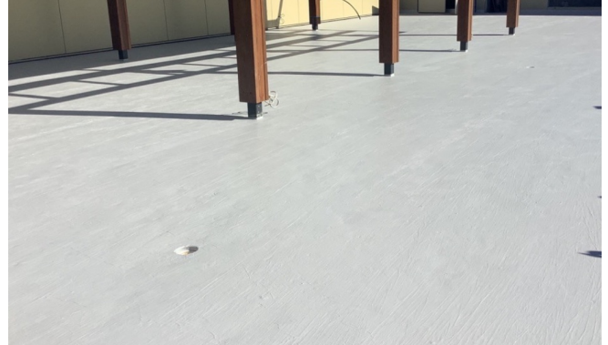
Pic 4. The substrate is clean
