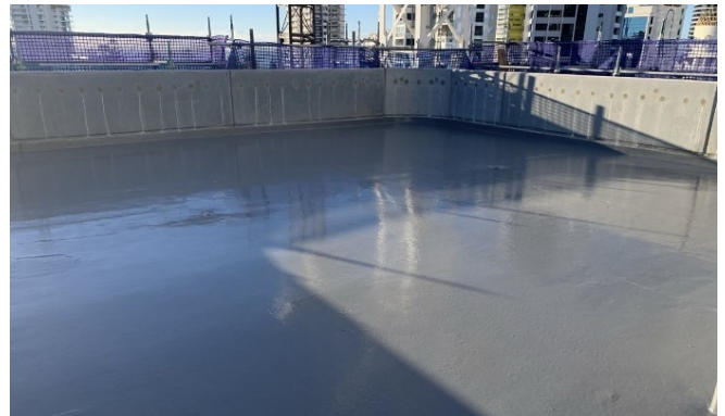
Pic 5. The membrane is applied at the correct thickness, preventing pinholes
