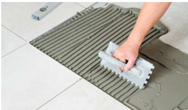
Pic 4. Cementitious floor application
