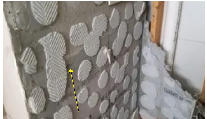
Pic 2. Spot bonding of tiles to substrate
