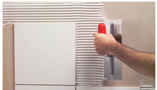
Pic 5. Mastic wall application
