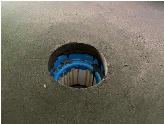
Screed to drainage flange is ready for waterproofing
