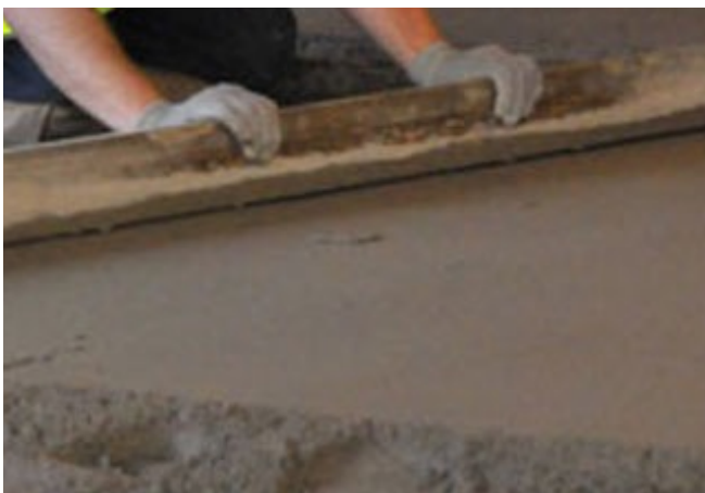
Take note of the thickness and consistency of the screed
